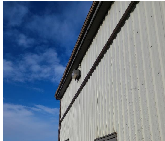
Singular light above the entrance. Unable to tell if it is LED light or not. More directional lighting would be recommended to be able to point down toward door and also outward into the yard.
